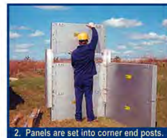
2. Panels are set into corner end posts.
