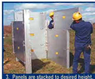
3. Panels are stacked to desired height.
