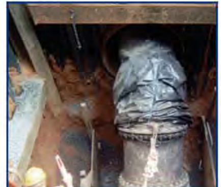
Sheeting around Bore Casing
