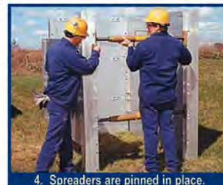
4. Spreaders are pinned in place.
