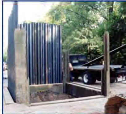
Guide Frame Tight to Excavation
