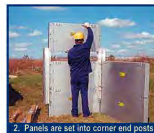
2. Panels are set into corner end posts.
