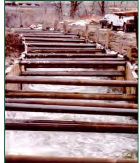
Spreader Set 5" Sch 80 - 4 Pipe "I"
