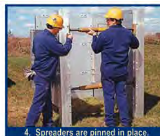
4. Spreaders are pinned in place.
