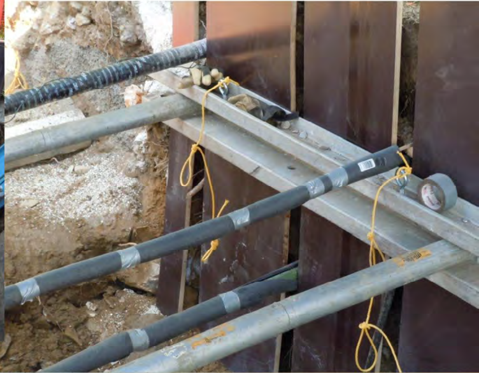
Top & Left: Aluminum Hydraulic Shoring with Finform
